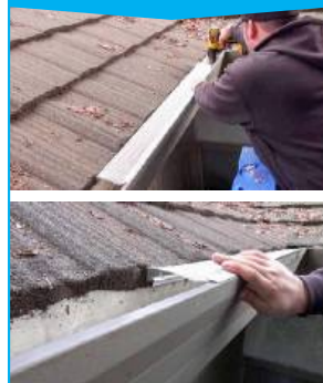
SOFT METAL ROOF
