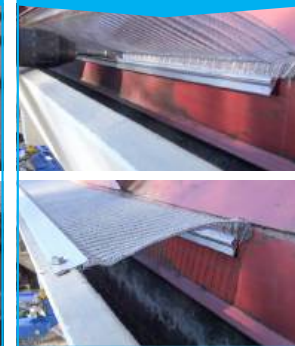
STANDING LOCK METAL SEAM
