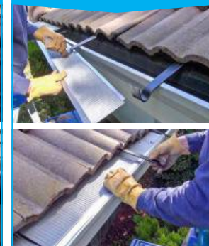
VILA TILE ROOF
